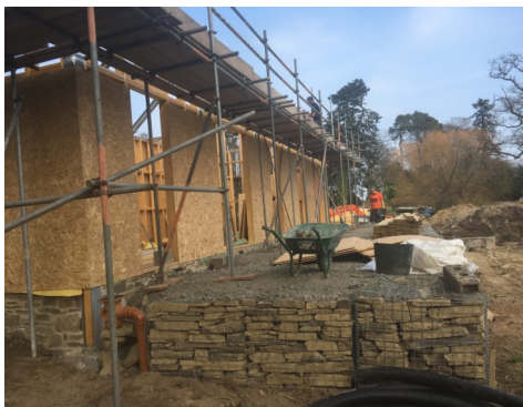
Southern facade showing gabions filled with local stone
